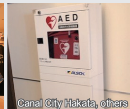
Canal City Hakata, others AED installation
